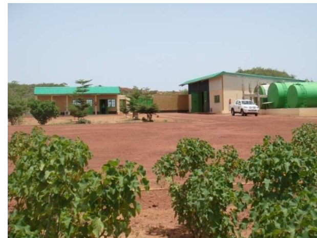
Biodiesel production Factory, Mali
