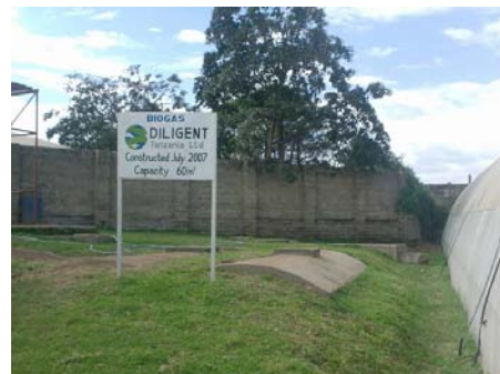
Figure 5-20 The 60 m 3 digester at Diligent Tanzania Ltd. (installed by Camartec, Arusha)
