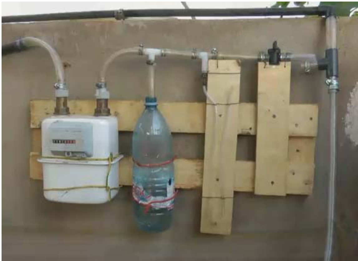
Figure 7-7 Gas meter, pressure relieve system, gas pressure meter, and main valve
