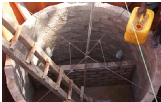
Figure 5-6 Constructing the separation wall
