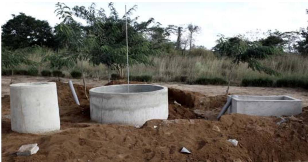
Figure 5-10 Inlet, reactor and outlet
