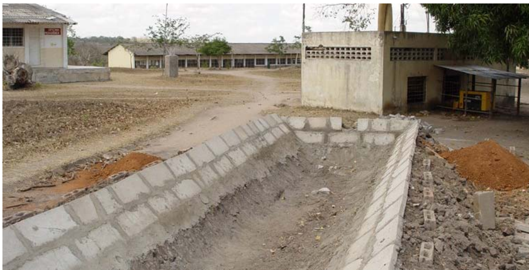
Figure 4-7 Placement of reinforcements for a 60m 3 digester
