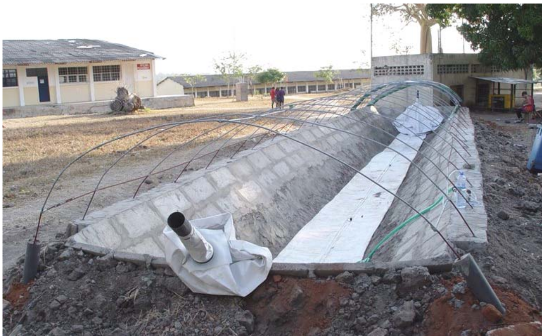
Figure 4-10 Digester bag ( 60\text{m}^3 ) placed inside the ditch
