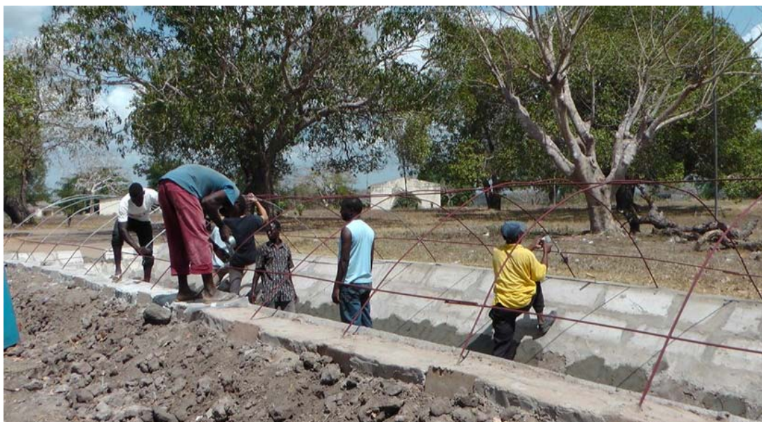
Figure 4-8 Roof construction of cement iron (60m 3 digester)
