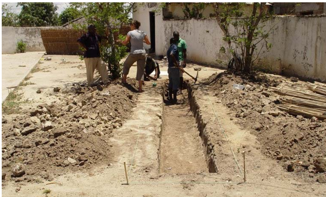
Figure 4-5 Excavation of a 6m 3 digester ditch
