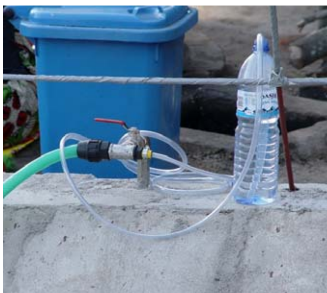
Figure 7-4 Pressure relieve system
