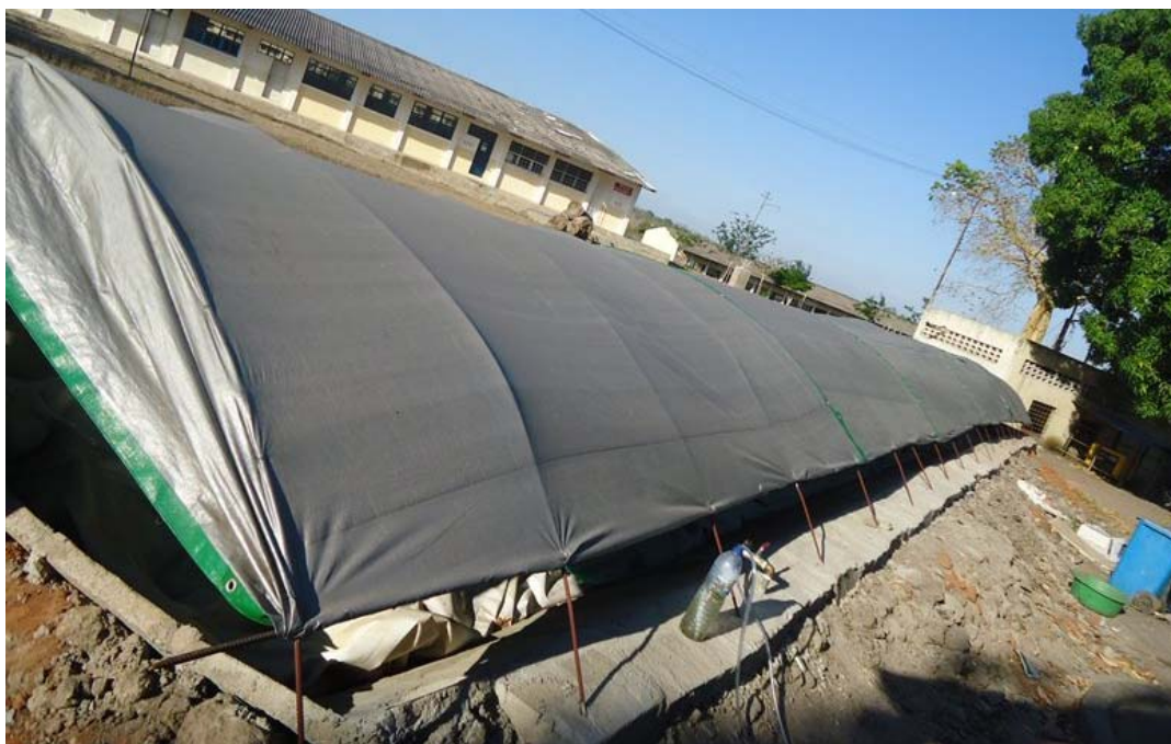
Figure 4-9 Roof cover (60m 3 digester)
