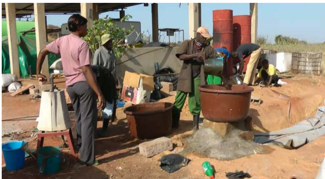
Figure 6-1 Filling of a 12m 3 digester
