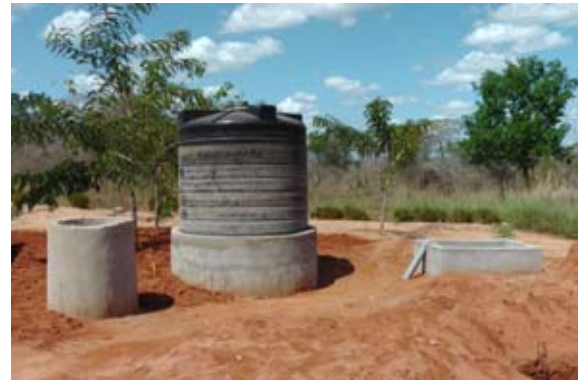
Figure 5-2 Floating dome system
