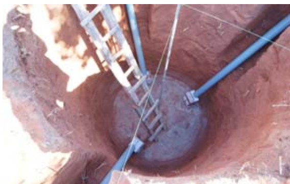
Figure 5-5 Reactor pit with 2 inlets and 1 outlet
