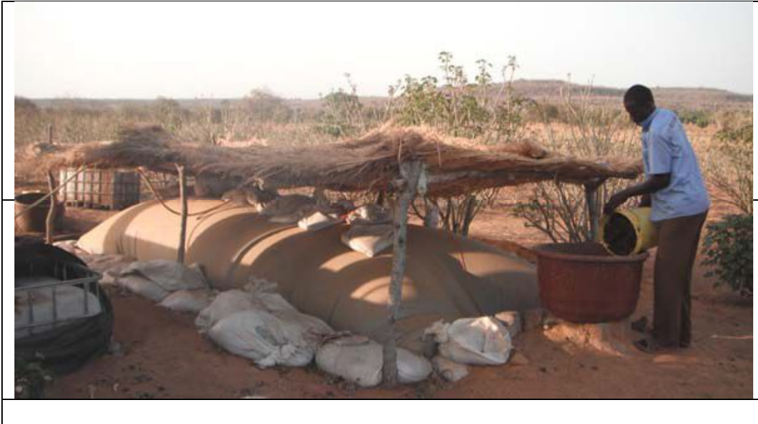
Daily feed of a 12 m 3 PVC plug-flow digester
