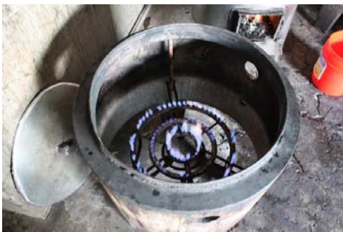
Stove run by biogas at Diligent Tanzania Ltd.
