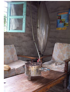
Figure 22: Biogas storage and cooker, Engaruka
