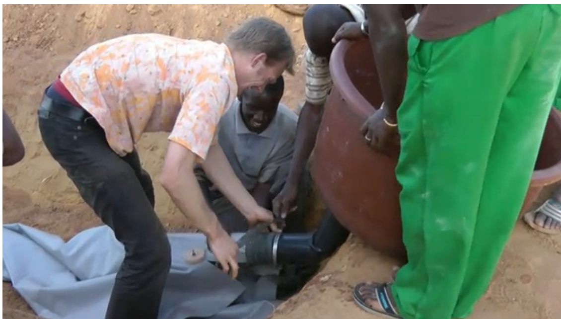
Figure 14 Placing the inlet pipe and bucket
