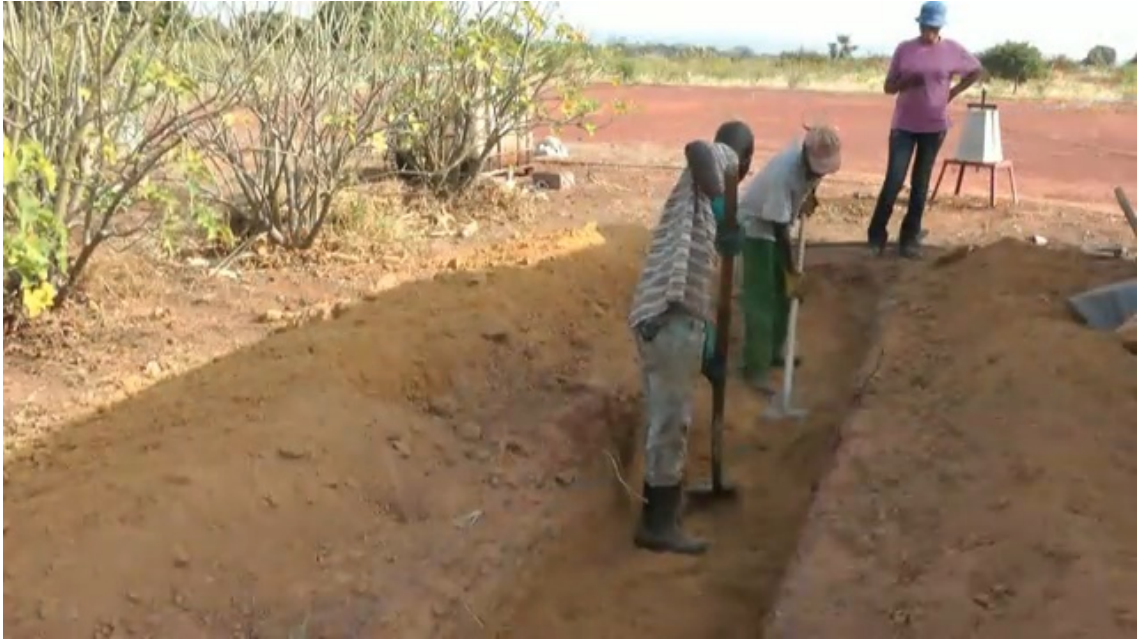
Figure 10 Excavation of a 12 m 3 digester ditch
