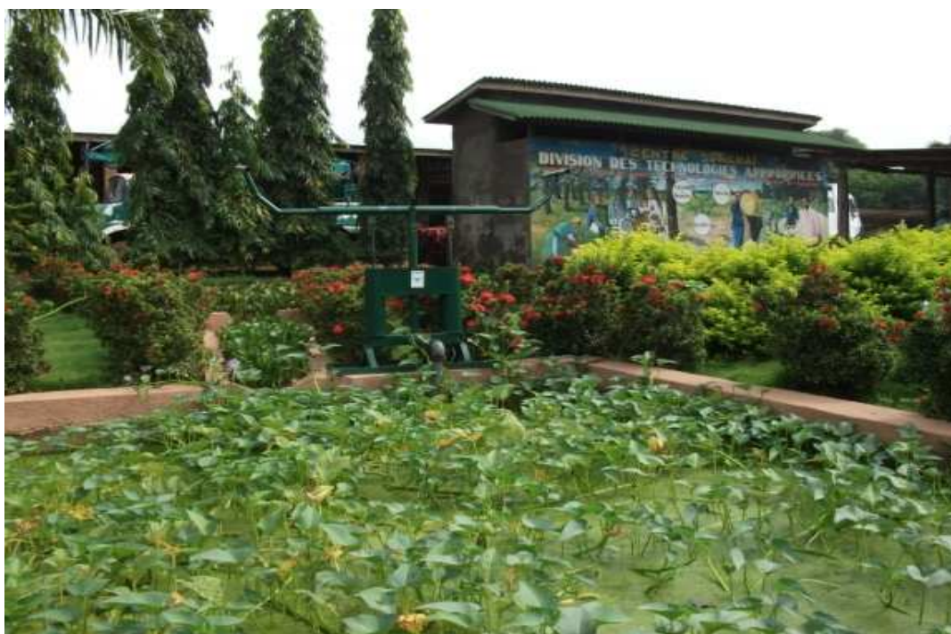
Figure 10: Water hyacinth ponds for wastewater treatment at the Centre Songhai, Porto Novo, Benin
