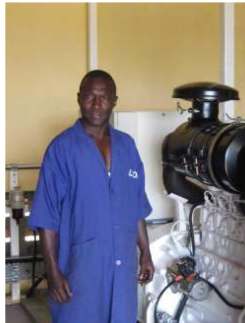
Figure 14 Technician standing in front of one of the Deutz generators, Garalo, Mali.
